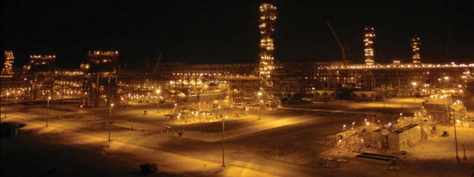
The Hawiyah NGL recovery plant (shown here in late 2007) at the Hawiyah gas processing plant near Ghawar oil field south of Dhahran is on track for start-up this year. Photograph from Saudi Aramco.
